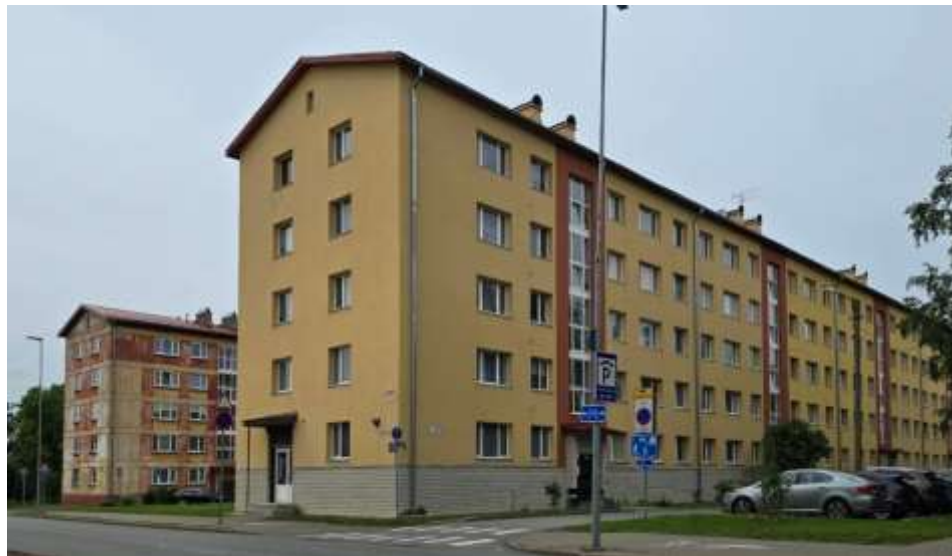
Figure 3. Renovated housing façade in Narva showing insulation and energy-efficiency improvements on the background of non-renovated building.
