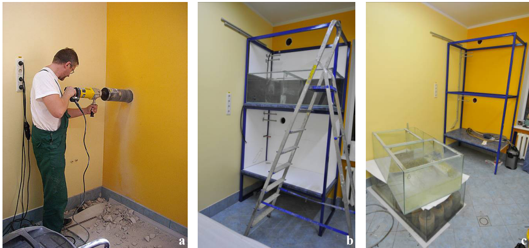
Fig. 1. Construction process of aquarium equipment for keeping D. latissimus ; a - preparing of ventilation apertures in the wall.; b - finished metal frame and central water supply; c - metal frame with styfoam insulation.
