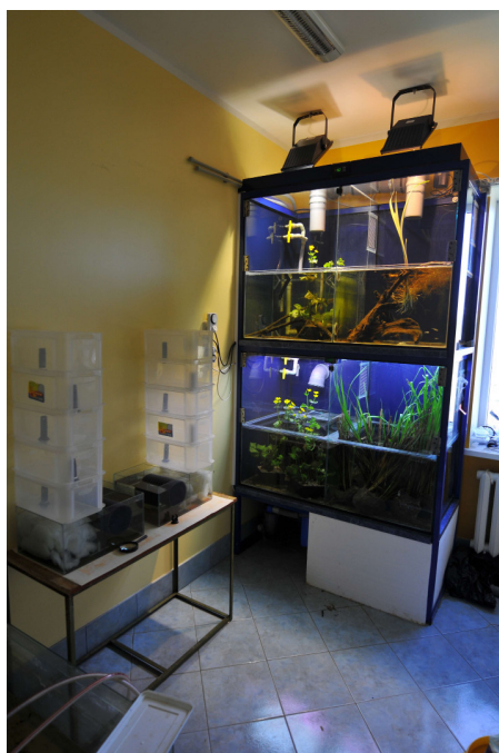
Fig. 9. General view of the ready aquarium installation with closed water supply for keeping D. latissimus (in spring-summer operational mode) ("Latgale Zoo", Daugavpils, Latvia).
