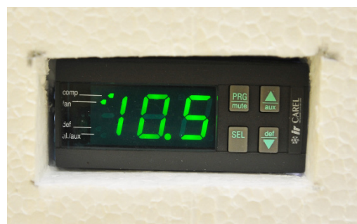
Fig. 5 Thermoregulator (Carel IR) in semi-season mode.
